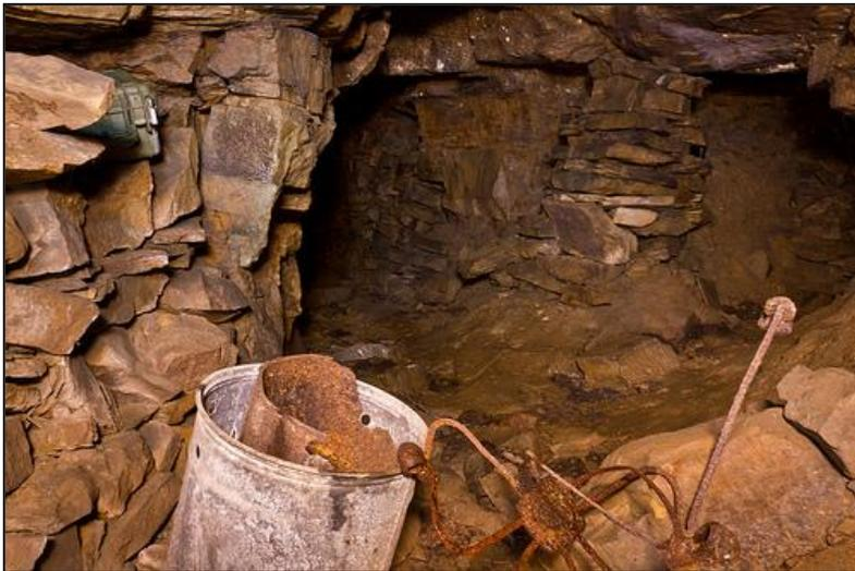
**Image 1** This image shows main tunnel intersection located approximately 7m in from the mine entrance. An Anabat recording device is shown in the top left of the image. A thermometer was installed on the dry stone support in the top right of the image.
