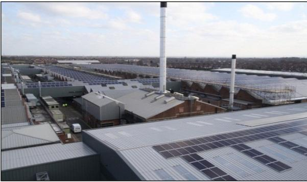
The Bentley Factory in Crewe built in the 1940s is ideally situated to generate solar power as the “saw tooth” factory roofs are south facing at an angle of 20 degrees. It is the UK’s largest rooftop solar PV array, owned and operated by solar power generator, Lightsource Renewable Energy and installed by main contractor Solarcentury.
