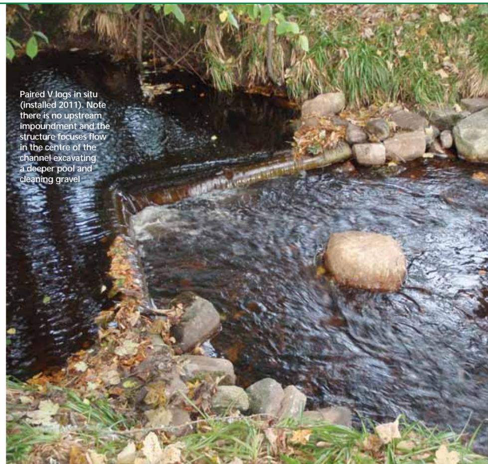
Paired V logs in situ (installed 2011). Note there is no upstream impoundment and the structure focuses flow in the centre of the channel excavating a deeper pool and cleaning gravel
