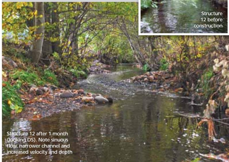
Structure 12 after 1 month (looking DS). Note sinuous flow, narrower channel and increased velocity and depth
