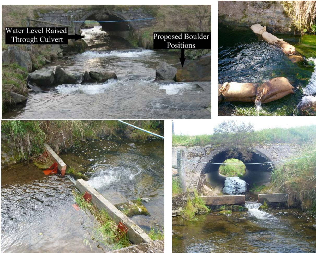
Figure 2 Culvert barrier modifications; (clockwise from top left); The original proposed modifications using boulders, The sandbags used in the trial, The finished beam installation on, and finally brackets holding beam in place. This work was funded by Patagonia.
