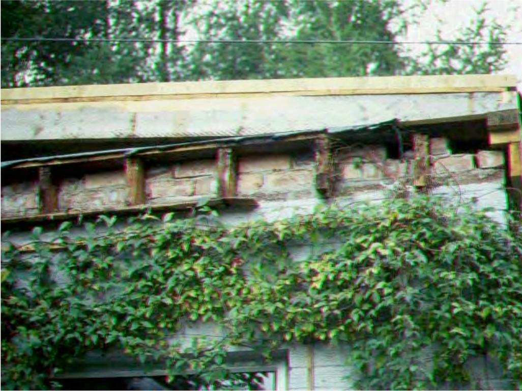
*Fig. 5.1* The exposed roof edge showing the joist ends
