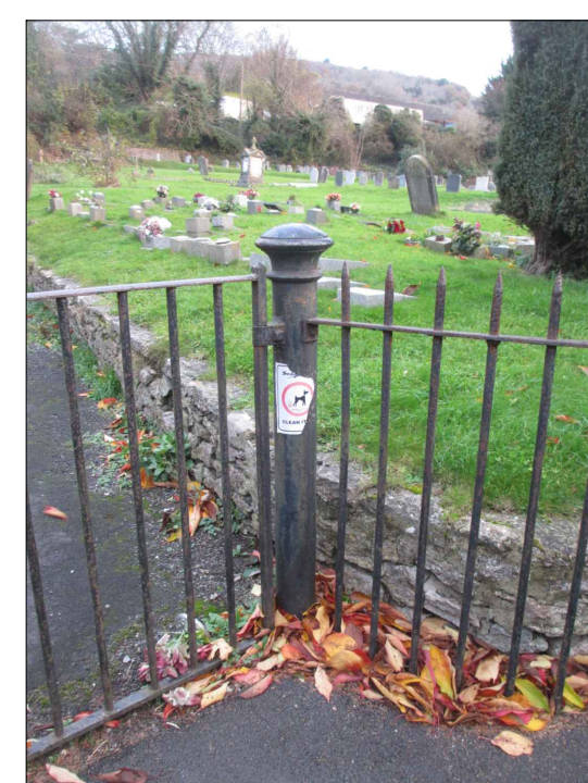
Photo showing existing post to terminate railings.
