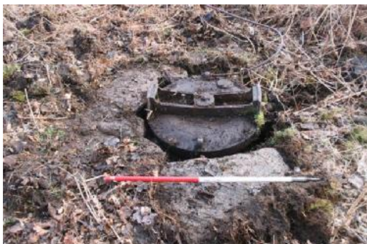
Achlorachan horse gang, gearing mechanism and shaft
